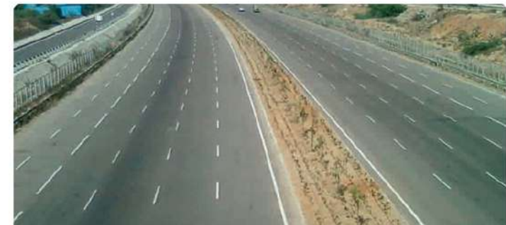
250 Meter Expressway of 110 kms connecting Ahmedabad - Dholera - Bhavnagar.
