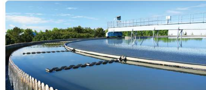
Water Treatment Plant - Tender has Been awarded to SPML of INR. 90 Cr. A water treatment plant of 50 MLD will be established.
