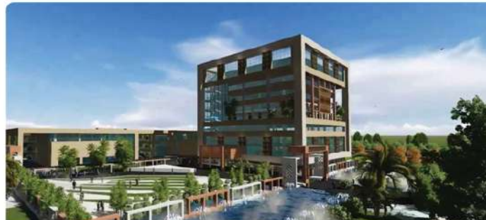
ABCD Building - Tender has been awarded to Cube Construction of INR. 72.31 Cr. Work at site is Completed.
