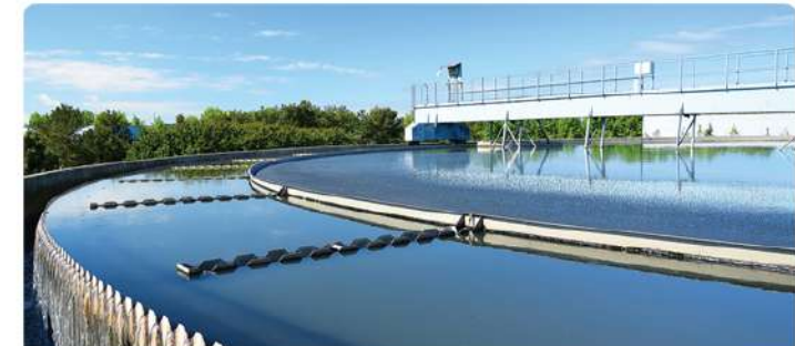
Water Treatment Plant - Tender has been awarded to SPML of INR. 90 Cr. A water treatment plant of 50 MLD will be established.
