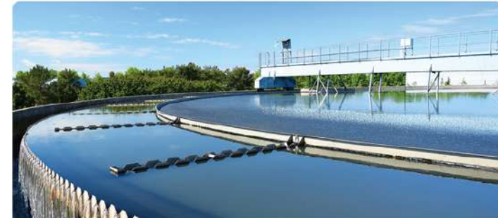
Water Treatment Plant - Tender has been awarded to SPML of INR. 90 Cr. A water treatment plant of 50 MLD will be established.
