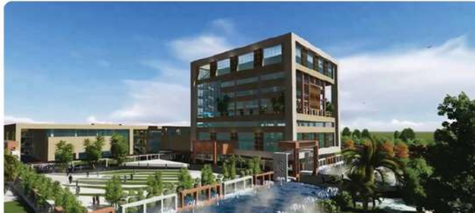
ABCD Building - Tender has been awarded to Cube Construction of INR. 72.31 Cr. Work at site is Completed.
