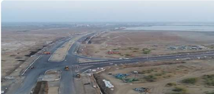
Roads and Services - Tender has been awarded to L&T of INR. 1734 Cr. L&T has mobilised on site & work has already commenced.
